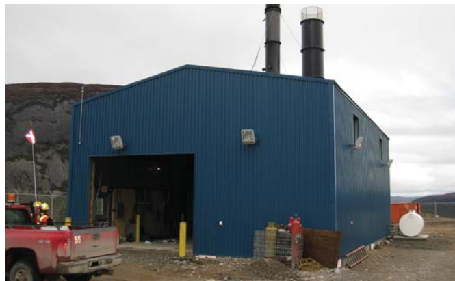
The new incinerator building at the waste transfer station. A new larger solid waste incinerator unit was installed and tested in 2009.
