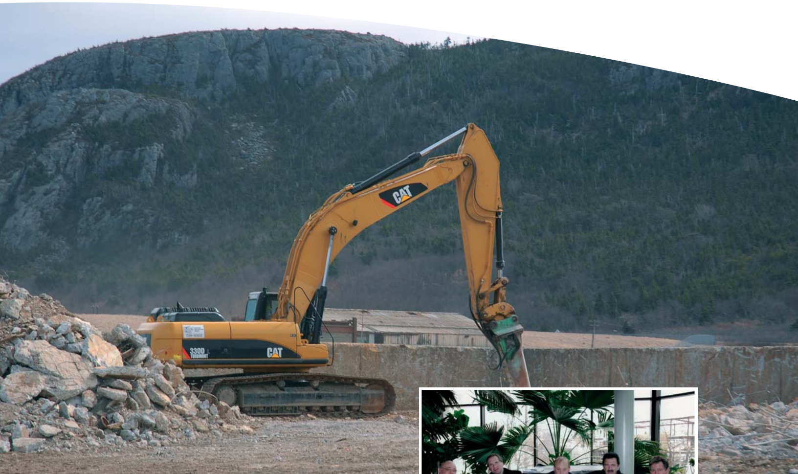
Demolition work at the Port Site in Long Harbour.
