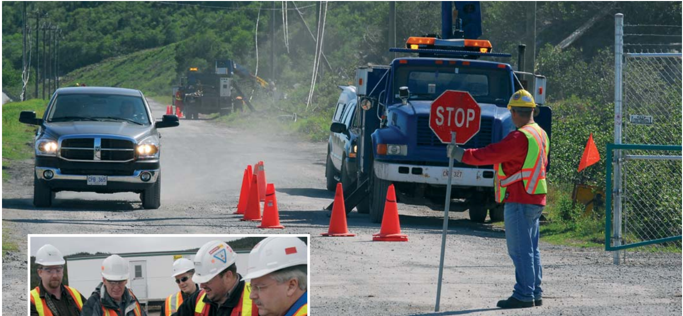
Temporary Power installation at Long Harbour Construction Site.
