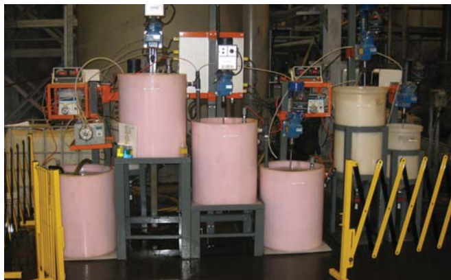
The pilot plant, located inside the concentrator building.
