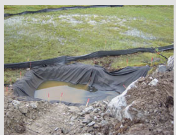
Silt fences prevent run-off from a settling pond into Camp Pond.
