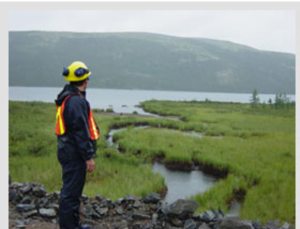
Labrador Inuit Association Environmental Monitor, Donald Lampe, checking culvert installation.
